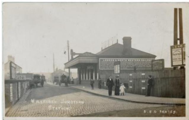
2751 Wilsden Junction railway station, exterior with carriages R/P (1) £18 - £20
